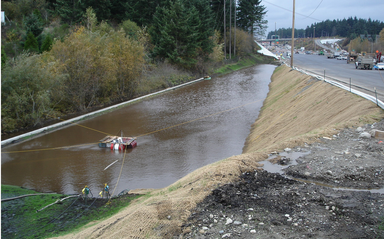
Figure 2 - 34. Floating Platform with Struts
